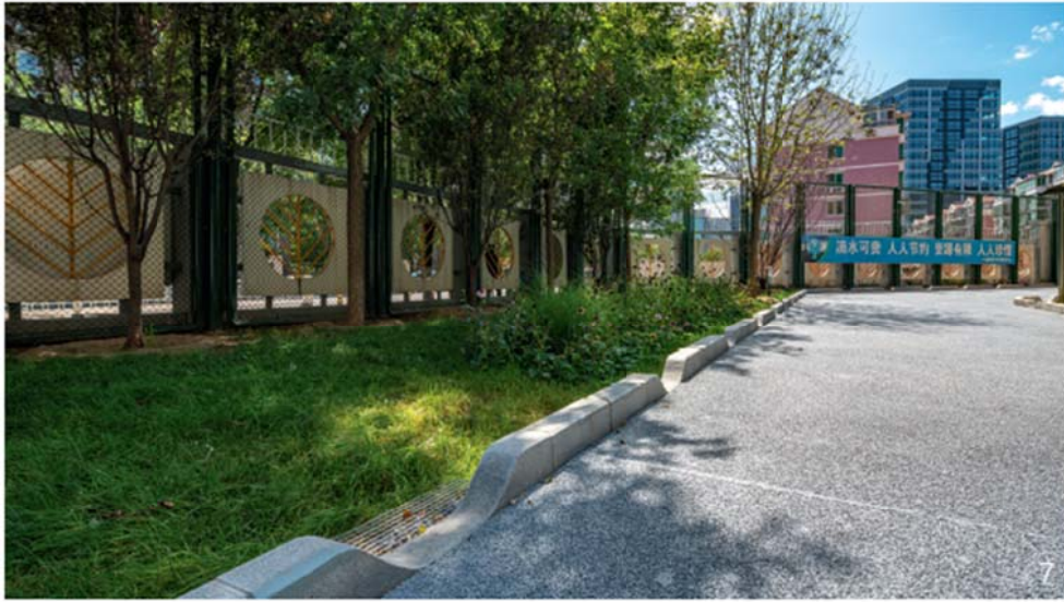
道路周边下凹绿地改造 Transformation of Sunken Green Space
