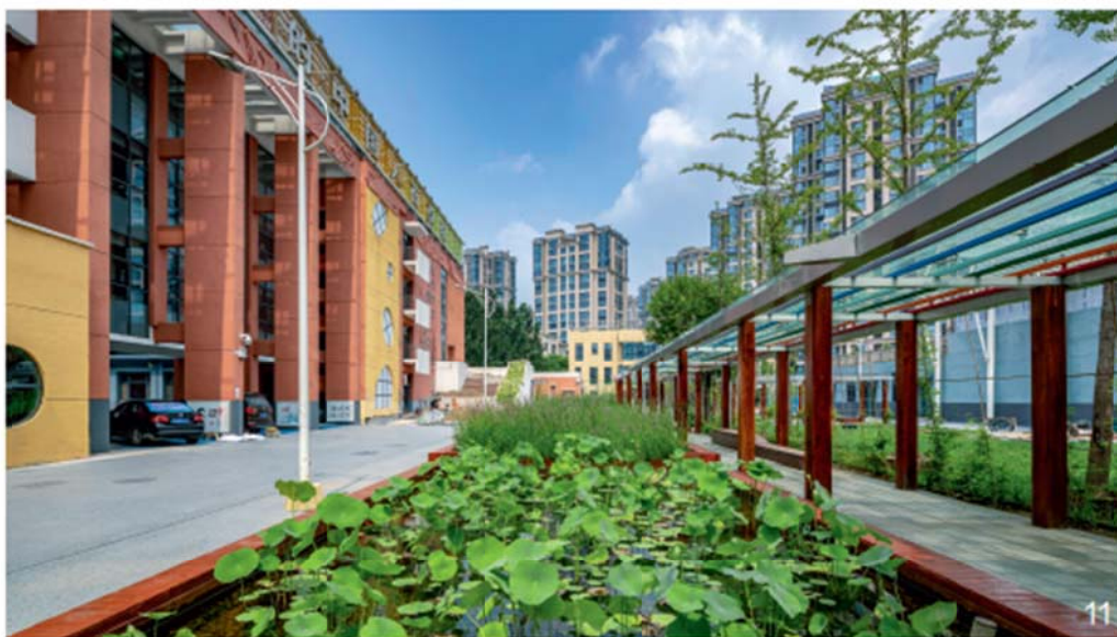
湿地长廊雨水处理系统 Rainwater Treatment System in a Wetland Gallery
